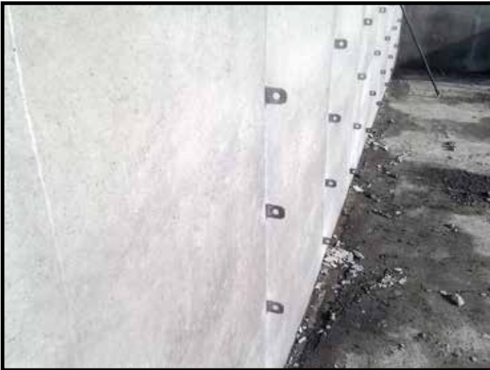
New Forms with the Pour Ready Process
